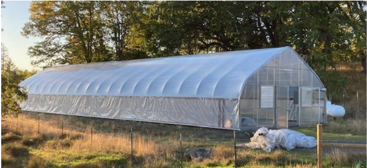
Greenhouse, New Dual Poly Installation, September 2023
