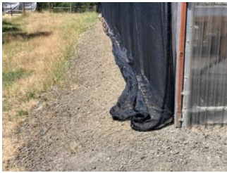
Site graded to drain away from production site.
